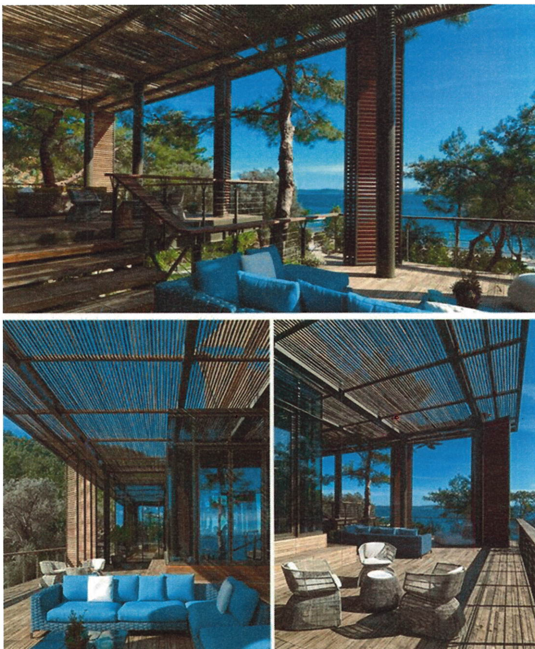
Figura 17 – Bodrum Demirbuku Houses Clubhouse
